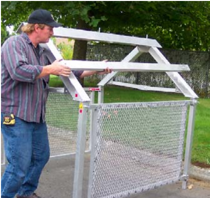
Attach the top truss connectors.
