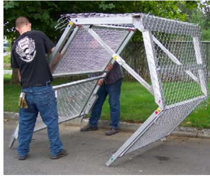
Attach the bottom side panels. These are color coded.
