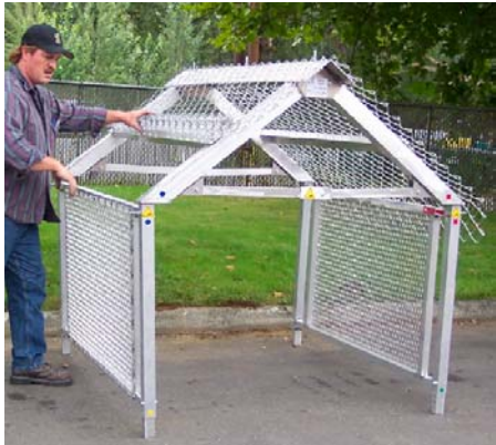
Roll the wire mesh across the top.
