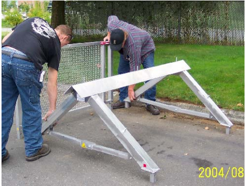
Attach the upper side panels. All are color coded
