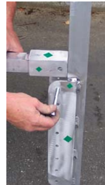
Insert bolts to each side.
