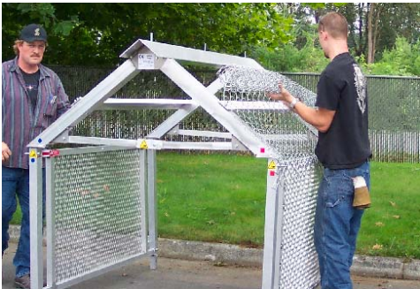
Roll the wire mesh across the top.
