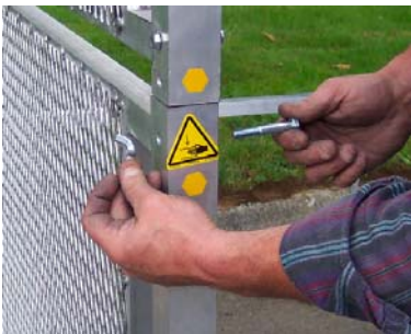
Insert bolts to each side.
