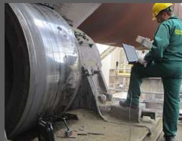
HOT KILN ALIGNMENT
